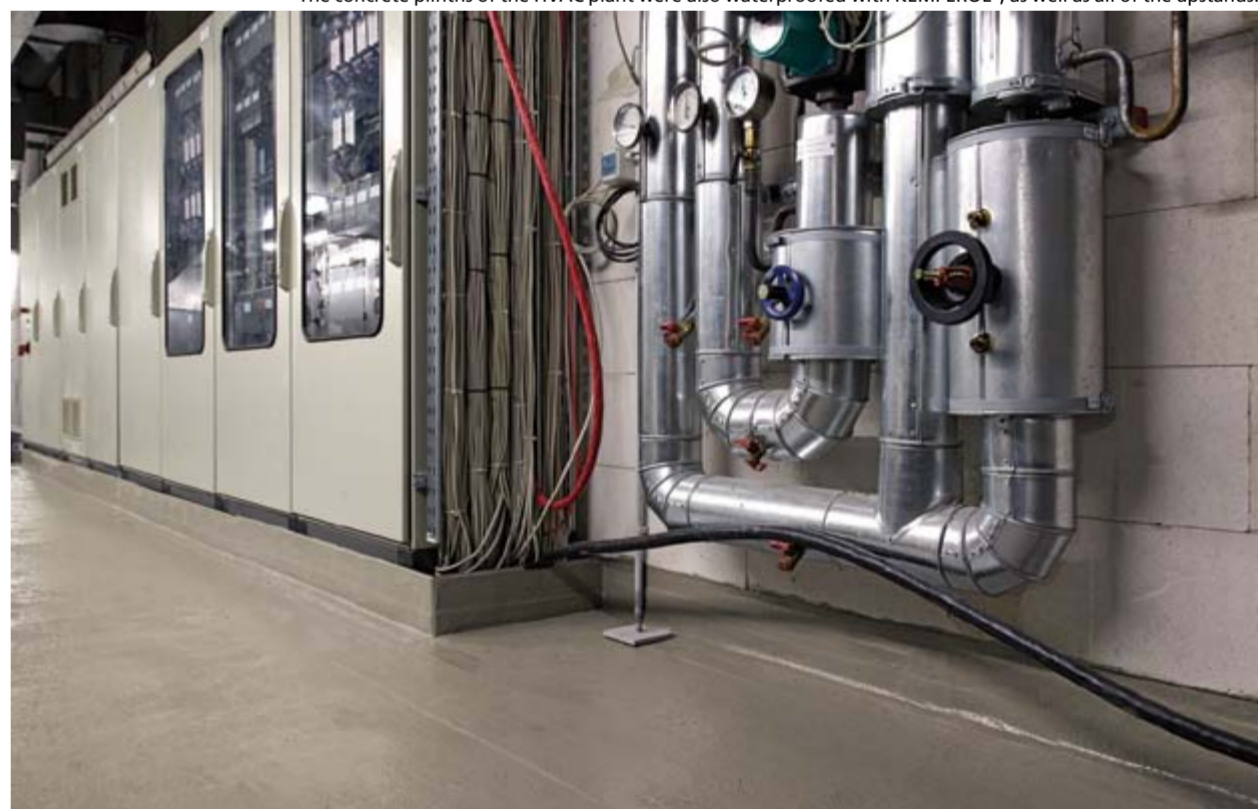
The museum exhibition rooms below the HVAC plants are protected by KEMPEROL® waterproofing. The concrete plinths of the HVAC plant were also waterproofed with KEMPEROL®, as well as all of the upstands.
